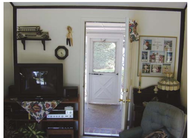
The porch door was replaced with windows so traffic is now directed to the front door. The floor in the porch area was raised to the level of the rest of the house.
